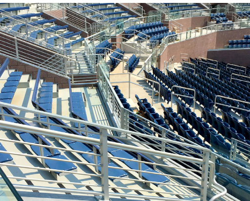
Horizontal Classic Picket Railing lines fan entrances, and front of fan seating areas of the new USTA Grandstand facility.
