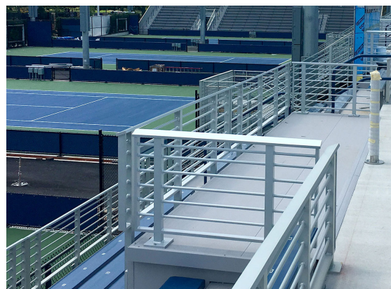
Anodized aluminum horizontal picket railing surrounds ADA seating areas at the newly redeveloped USTA South Campus.
