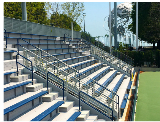
Top mounted horizontal picket railing line fan entrances to South Campus seating with Gridguard railing bordering bleachers.
