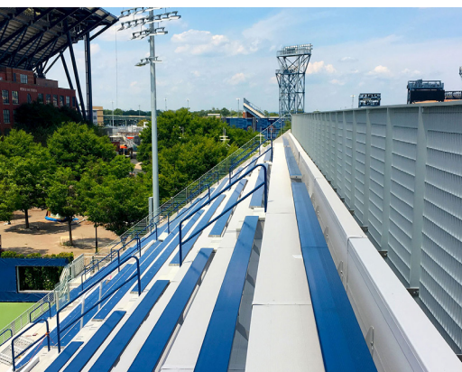
Side mounted Gridguard Railing with grated infill lines the back of the seating area on the USTA South Campus seating bleachers.
