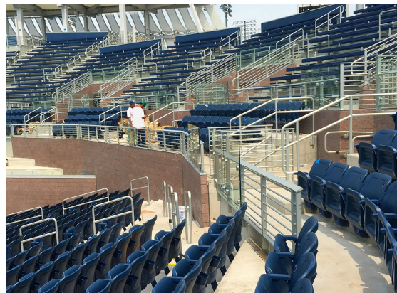
Top and fascia mounted glass railing can be found at the front of fan entrances and aisles at the new Grandstand.
