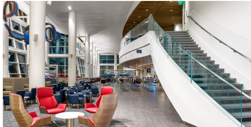
Glass railing with a flat bar stainless steel handrail is ideal for curved overlooks.
