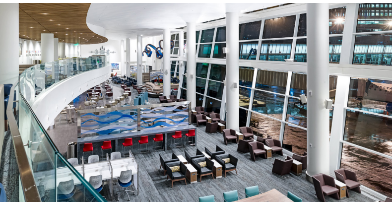
Track Rail is attached to a steel plate with through-bolts, creating a secure – yet sophisticated – second-story landing. Clear, tempered, laminated glass with EVA interlayer enhances the airy aesthetic.
